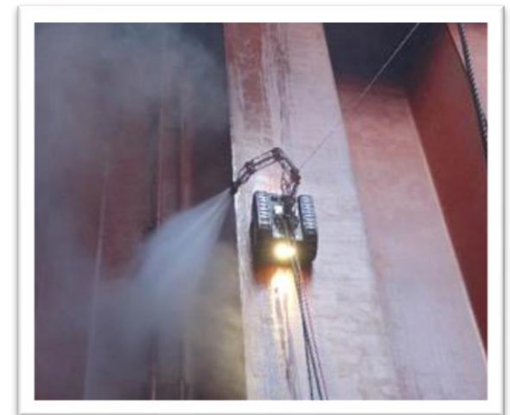
(Robot that washes high pressure water in the hold of our managed vessel)
