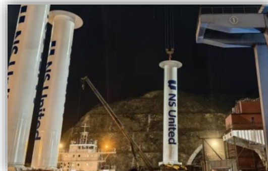
(Installation Work in Progress)
