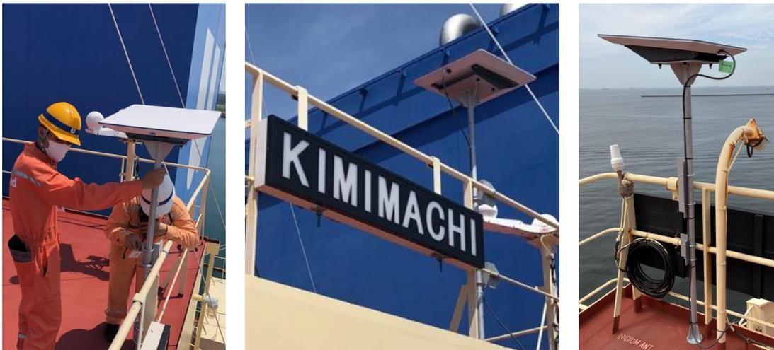
Installing antenna on board of a vessel
